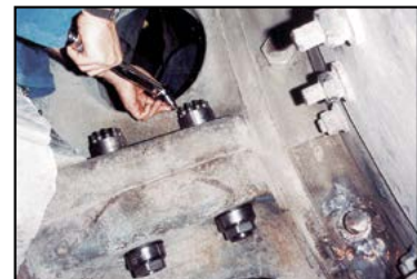
Split gear segment on rotary kiln.
