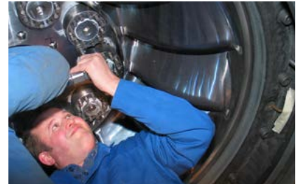
With Superbolt tensioners, joints in awkward positions in confined spaces can be tightened. This Francis wheel has regular maintenance requirements which became manageable with MJTs connecting the wheel to the shaft.
